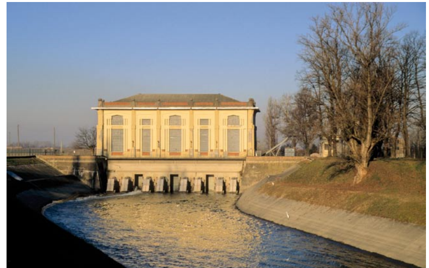
Santa Bianca, water works
