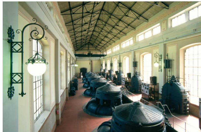
Argenta, Sairino Water Works
